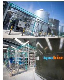
The project was developed by British firm Aquabio in 2016. The wastewater recycling plant is placed next to the food processing facility. Wastewater from the food processing facility is treated to potable water standards for reuse in the factory for all processes.
